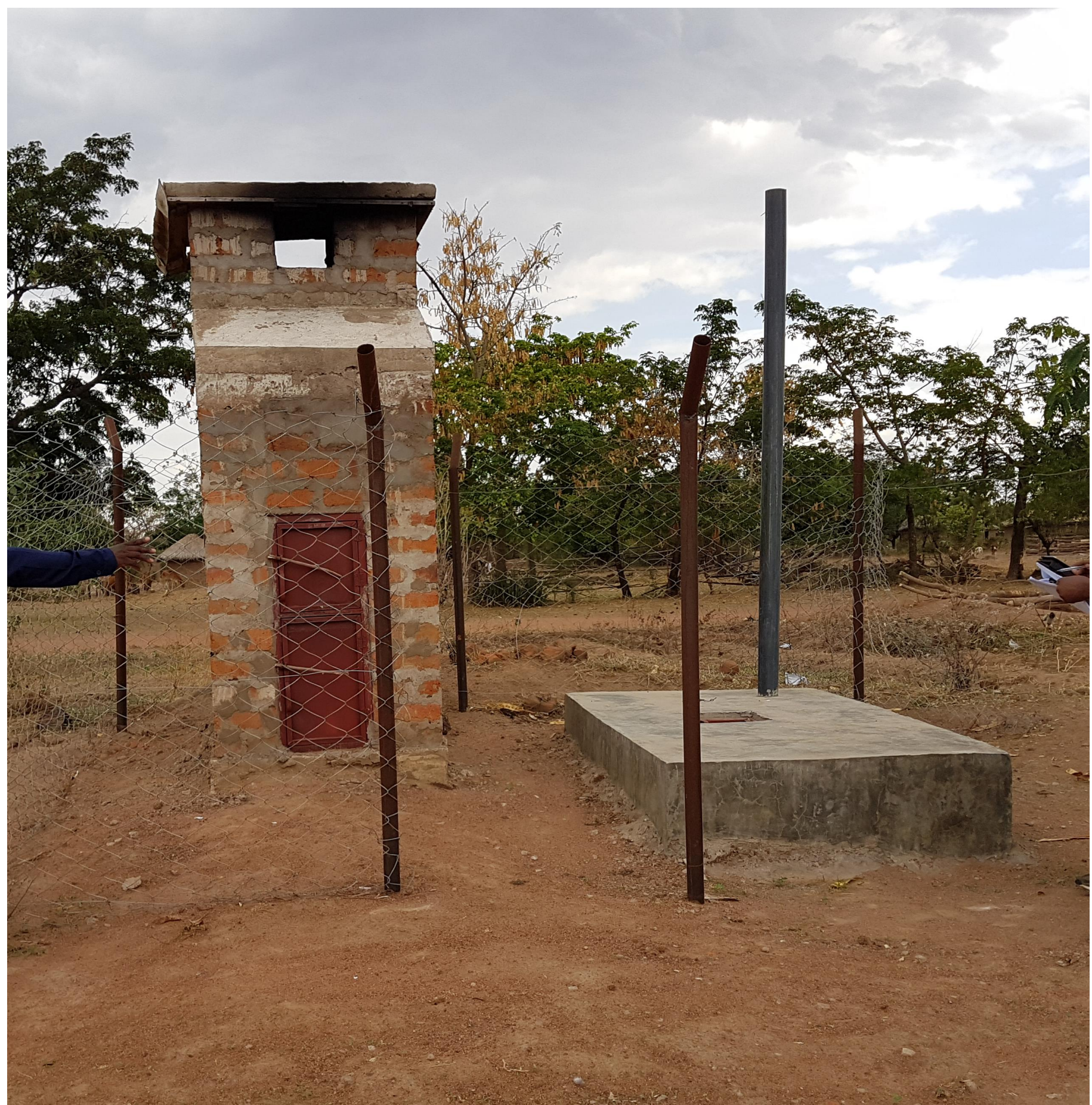
Fig. 1 Example of incinerator (left) and placenta pit (right) seen in Misungwi District
